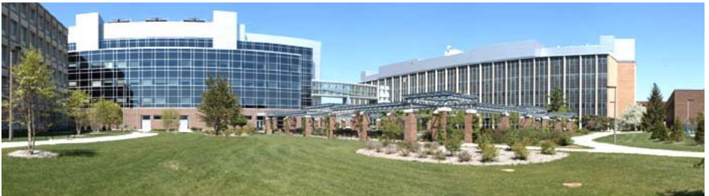
View of Biochemistry, BPS, and Chemistry from the newly finished courtyard. Pictures provided by Neil Bowlby
