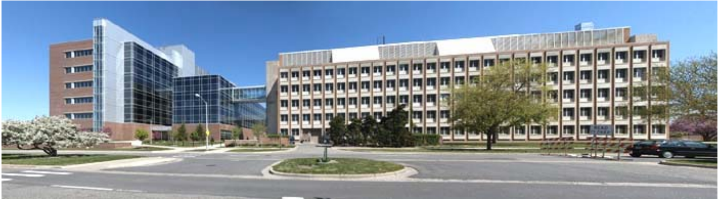
View of Biomedical and Physical Sciences and Biochemistry buildings from Wilson Road.
